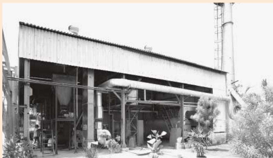
Hot Air Generator using environment friendly fuel (corn-cob)
