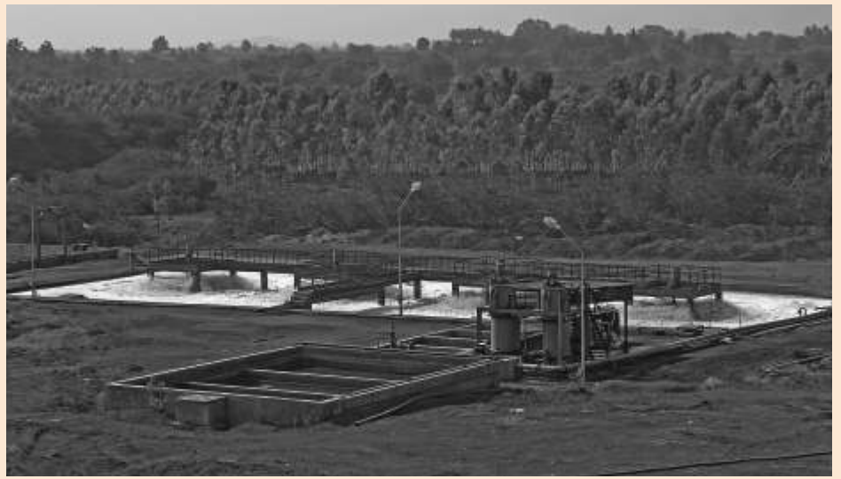
Effluent Treatment Plant
