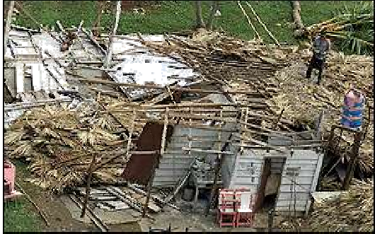
Hurricane Michelle damage in Cuba
