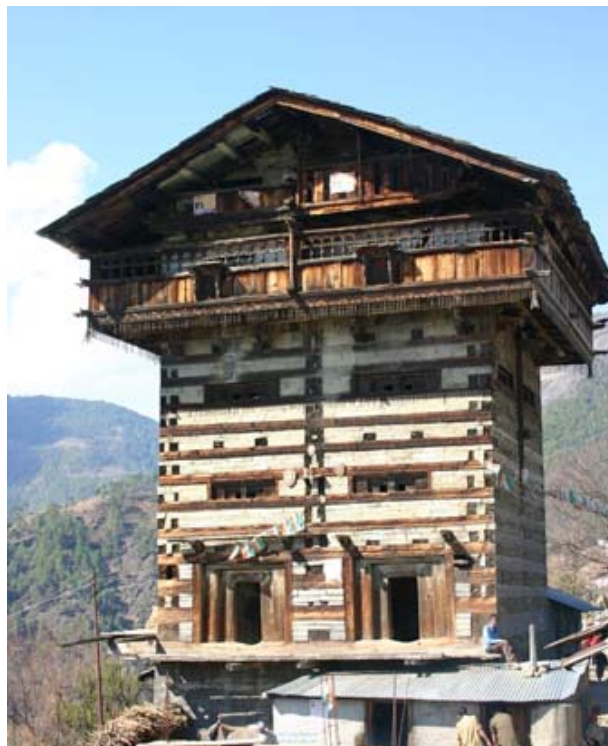
Figure 3. Five-storied structure of Koti Banal architecture constructed 880 ± 90 yrs BP.
